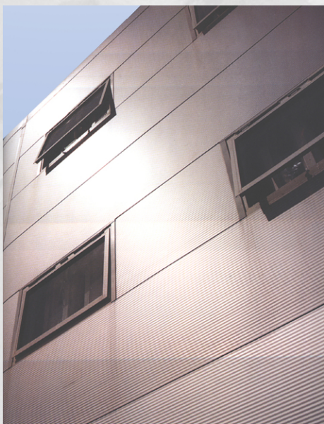
HOUSE BLOCK CLADDING DETAIL
